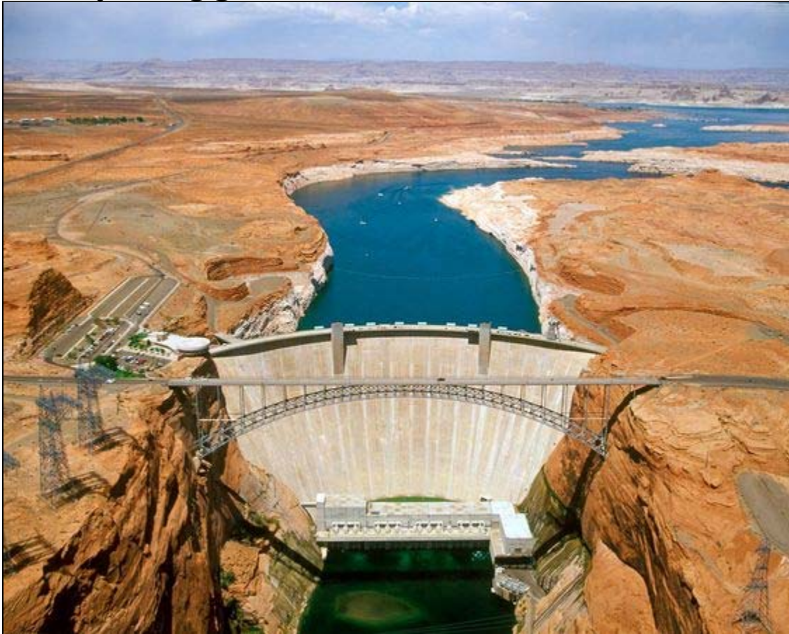
Aerial view of Glen Canyon Dam on the Colorado River in Page, Arizona.
